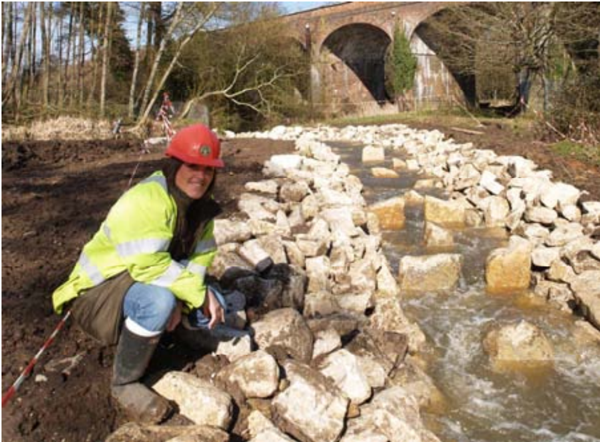
Fig.(14) The Botley Mill fish pass has opened up the River Hamble for the first time in hundreds of years.
